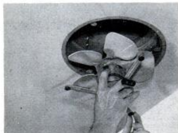
Below, reducer capping top of housing takes standard 8-in. furnace pipe to vent fan through roof as in drawing at right. The reducer has back-draft damper
